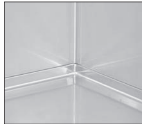
Detail of radius corner and tanked bottom
